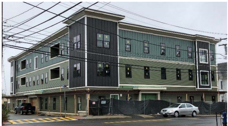
68 South Street - After
