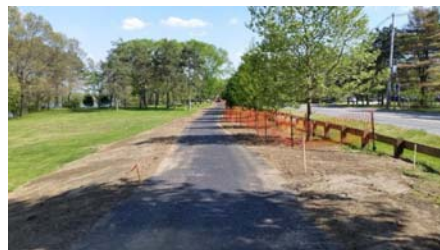
Dudley Road Multi Use Recreation Path nearly complete
